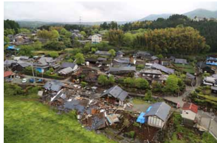
Destroyed Districts in Nishihara Village.
