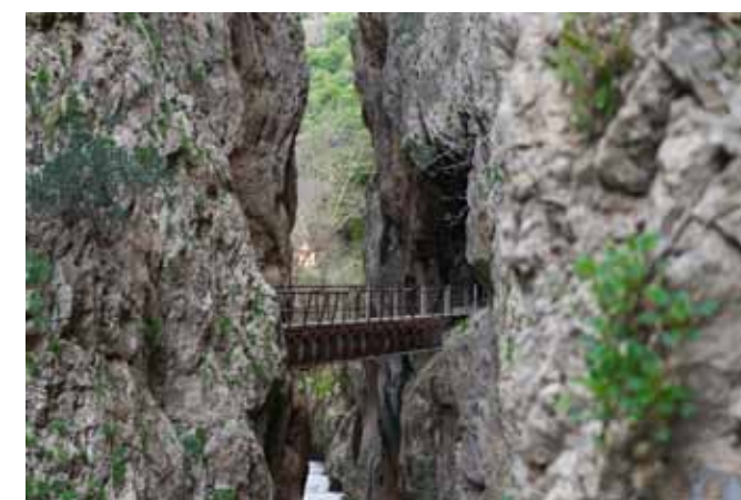
Vouraikos Gorge at Geosite Portes-Triklia, which according to mythology Hercules himself was responsible for its creation. The famous Odontotos rack railway crosses the steep slopes of the limestone in the gorge which have been uplifted by tectonic movements and sculptured by river erosion.
