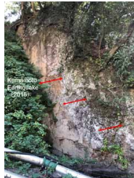
Futagawa fault. The vegetation attached to the rock decreases toward the left of the photo, indicating that the fault has moved repeatedly.
